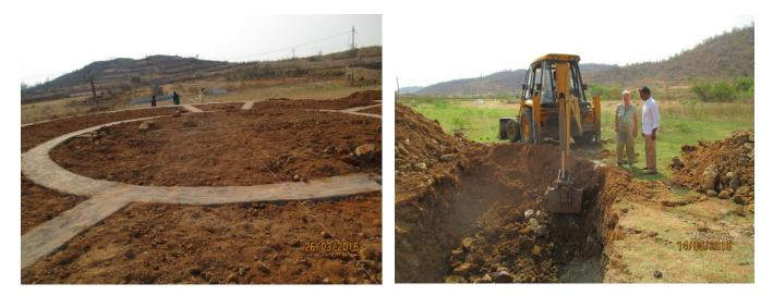
At present the foundation for the bear rooms is complete including the digging of the moat around the bear compound. It is 7ft deep and with the black stone slabs to cover the side and an additional wall of 5 ft, high the 12 ft straight wall will prevent the bears to escape.
