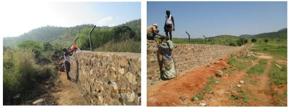
At present, 2-4-2016 the compound wall built with rough stones and cement is almost finished, 1.2 km long.
